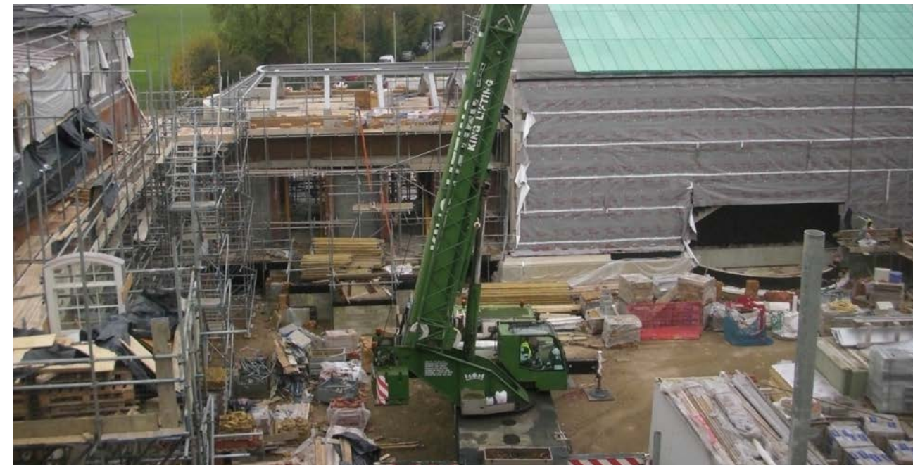
Construction of the Jafar Building
